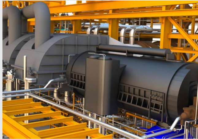
Fig. 2: Examples of CPP parts that could be reused for NPPs; a CPP turbine rotor (left) and a render of its outer casings (right) are shown (courtesy of Eskom).
